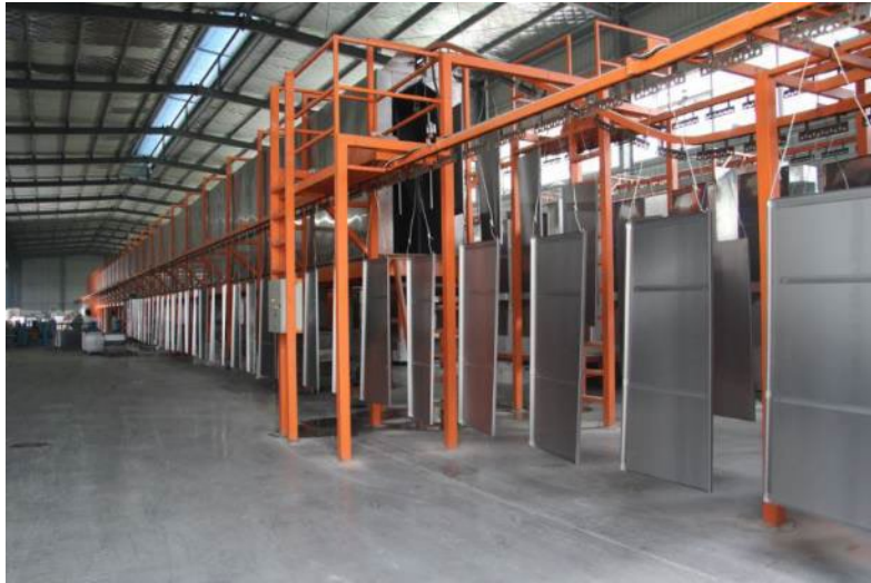
500-meter Germany Powder Coating Line
